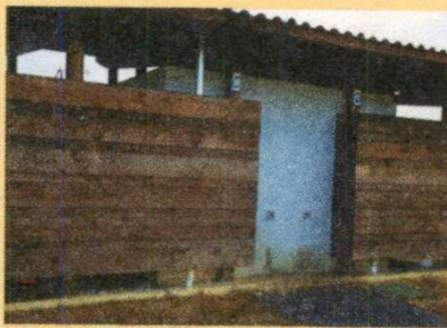
Shower houses at the Summit are built of locally harvested lumber.
